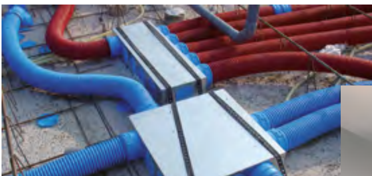
Suggested layout showing right-angle/straight air distribution manifold with 400 x 400 mm extractor plenum 00
