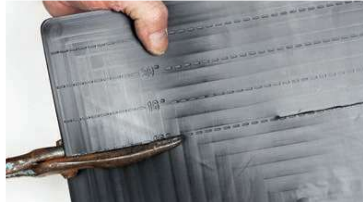
Step 2: As a guide, slate sizes are marked on the SolarFlash.
