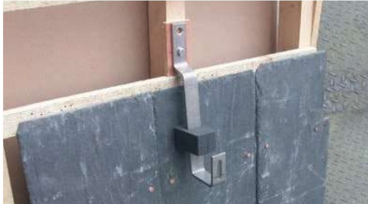
Step 1: Fix foam to bracket drop.
