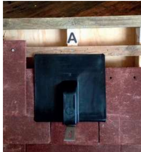
Step 2: Put SolarFlash (small) on the bracket.
