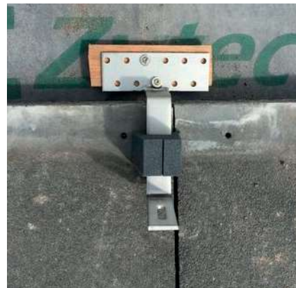
Step 2: Put SolarFlash (small) on the bracket.
