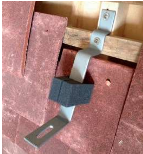
Step 1: Fix foam to the bracket drop.
