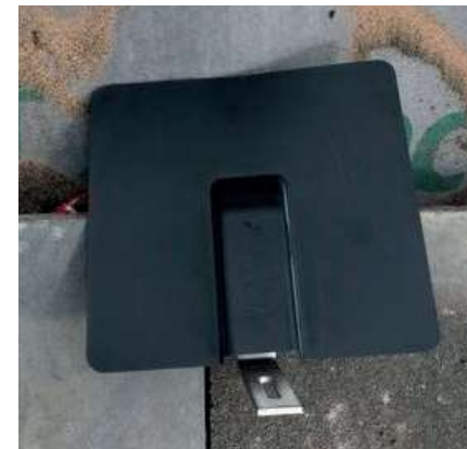
Step 3: Cut tiles around the hood of the SolarFlash as per page 12.
